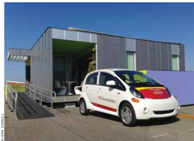
Above: The fluxHome, by the University of Southern California team, positions windows and doors to catch southern California’s southwest breeze. A large, centrally placed skylight acts as a solar chimney.
