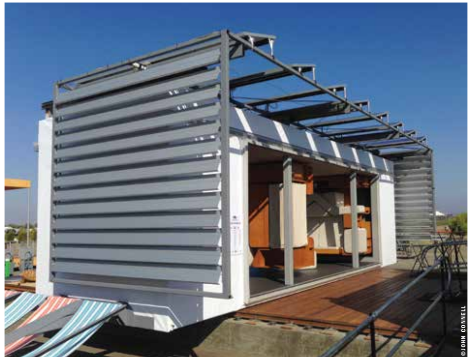
Top right: Third-place decathlon winner—AIR House, by the Czech Technical University team—has a passive solar canopy consisting of wood slats that cover the entire building and southern-facing wall and help eliminate the need for air conditioning.
