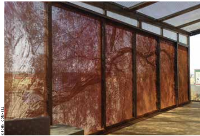
Above: DesertSol, by the University of Nevada at Las Vegas team, used a variety of passive energy strategies, including this metal solar screen, which was rusted to match the home’s weathered facade. It doubles as an artwork, embedded with the shadow of a mesquite tree.
