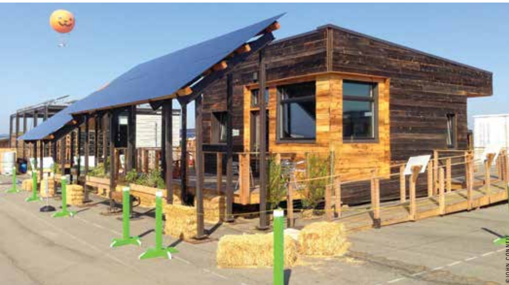
Above: The fluxHome, by the University of Southern California team, positions windows and doors to catch southern California’s southwest breeze. A large, centrally placed skylight acts as a solar chimney.
